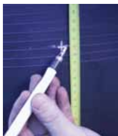
Mark the height of the centre of the additional connection
