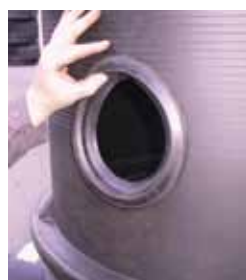
Install the inlet gasket
