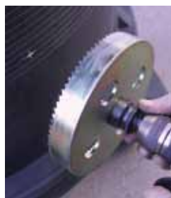
Drill a hole for the inlet gasket
