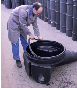
Attach and lubricate the gasket
