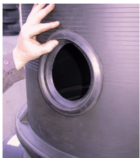
Insert the KS inlet gasket
