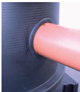
Connect the PVC pipe
