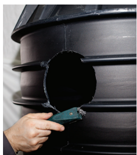
Clean and lubricate the rim
