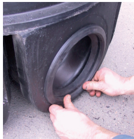
Install the inlet gasket
