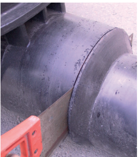
Cut off the extension
