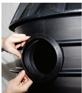
Insert the LKS inlet gasket
