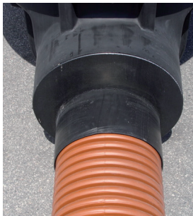
Properly lubricate the interior of the connection and the gasket, push the pipe into the chamber
