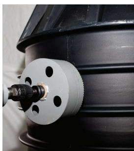
Drill a hole for a LKS inlet gasket
