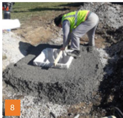
8 Preparation and concrete foundation levelling for the RC ring with a cast iron cover.
